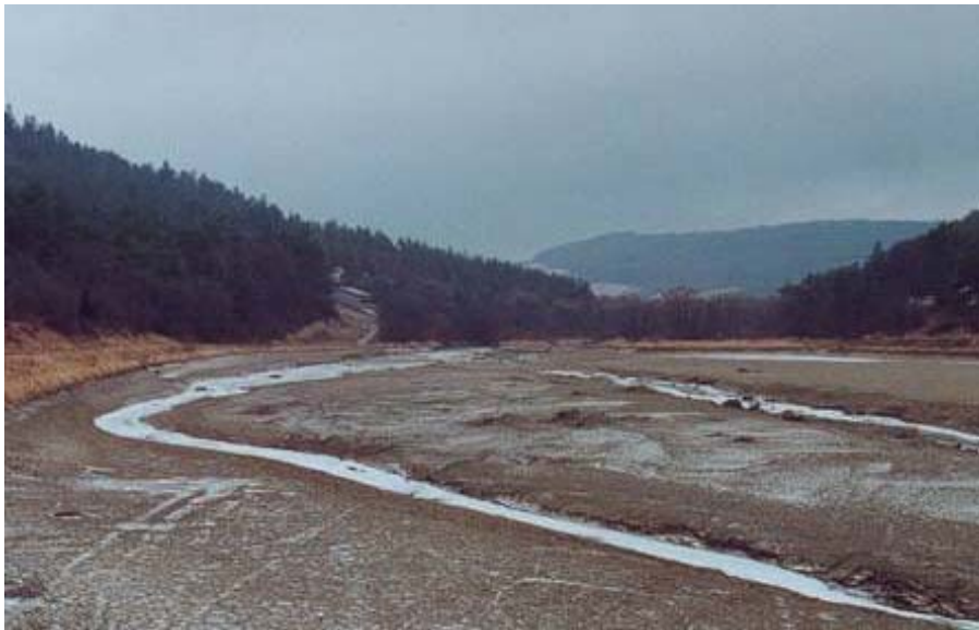
Fig. 3. Reservoir at Krempna – reservoir in winter. Photograph taken in 2002
