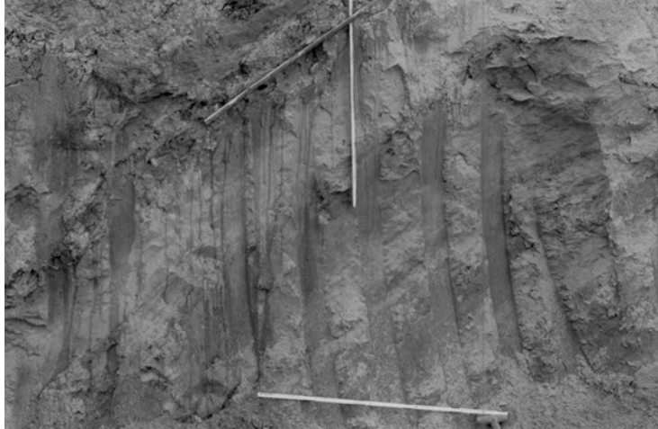
Fig. 2a,b. Pliocene clays in the Warsaw underground's tunnel (b – sharply outlined glaciotectionic dislocation)
