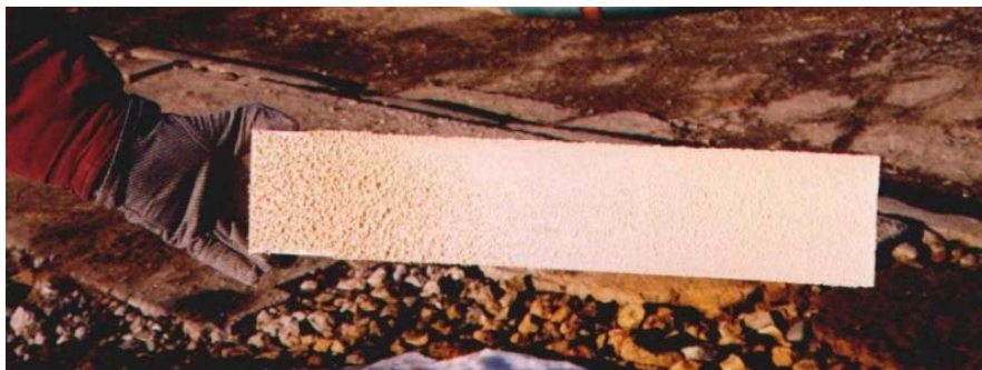
Figure 3. Deposit control plate after taking out from the recuperator
