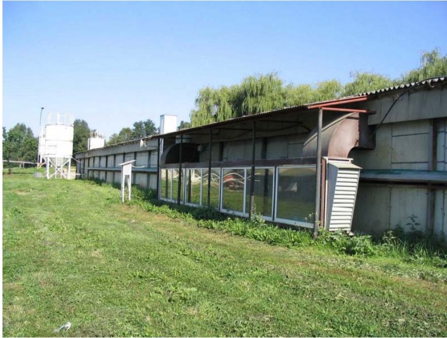
Figure 2. View of recuperator mounted in the broiler house in Ujazd. On the left, solarimeter and weather house for measurement of external air temperature and humidity
