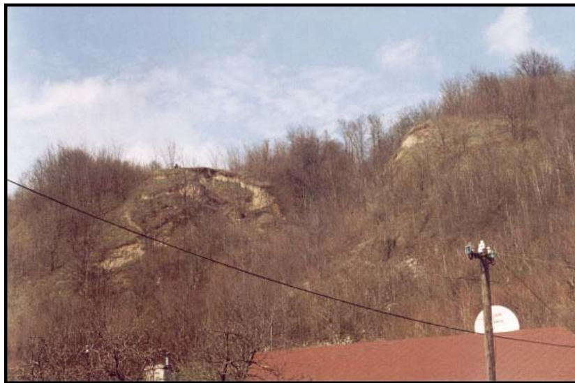
Photograph 1. The existing landslide in the Grodarz stream watershed
