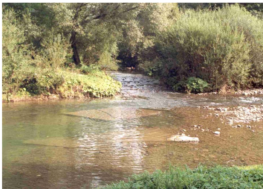
Photo 4. Łostówka - Mszanka confluence. Concrete platforms from devastated basin of concrete step after-toe built in Łostówka watercourse (photographed by M.Zygula)
