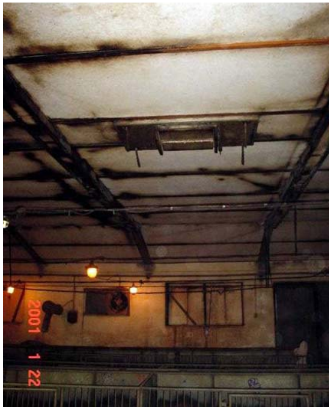
Figure 4. Impermeable ceiling consisting insulating panels PW3/A with high speed ceiling air inlets
