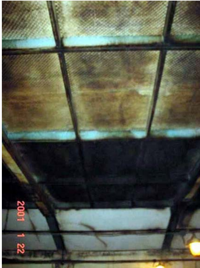
Figure 4. Impermeable ceiling consisting insulating panels PW3/A with high speed ceiling air inlets
