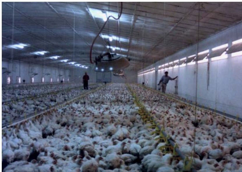
Fig. 5. General view of the building with 2 side walls visible with upward/downward air inlets in one wall and exhaust fans at the other
