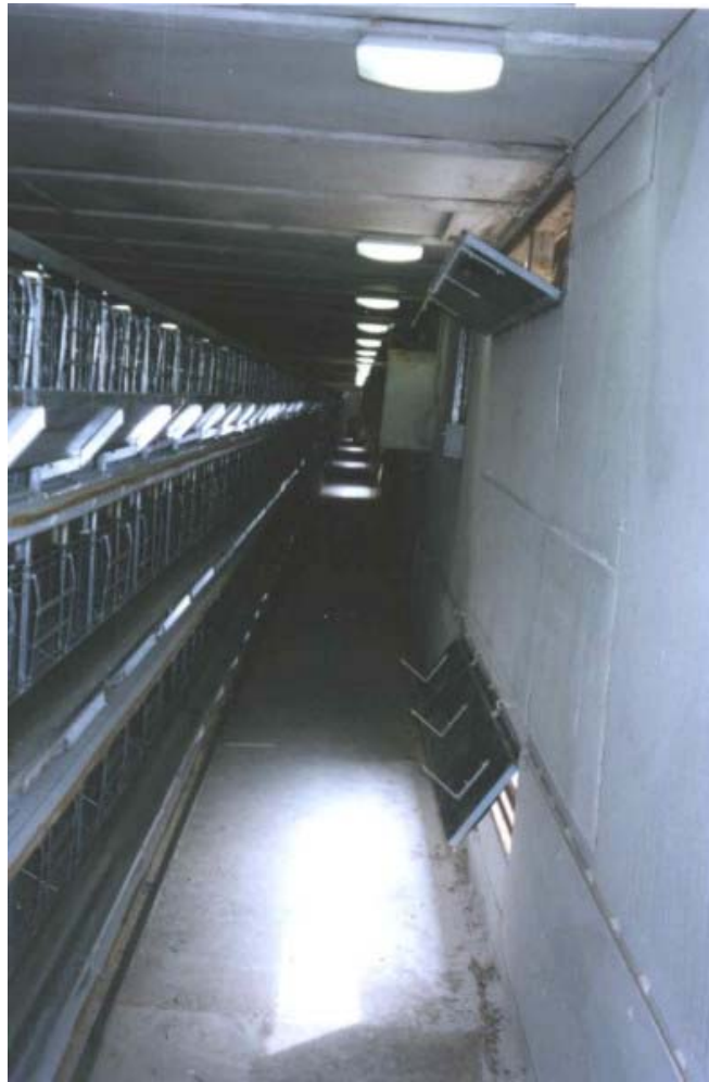
Fig. 4. Laying hens barn with separate air inlets for cold and hot weather
