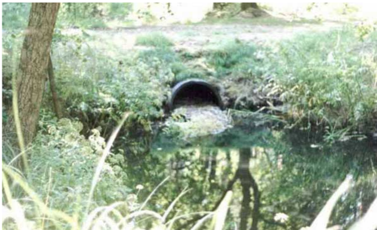
Picture 1. View of a road pipe culvert with the delaying elements
