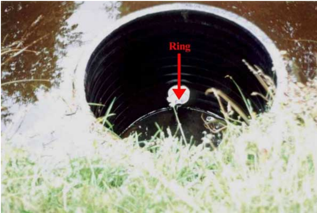
Picture 3. View of a limiting ring from a road pipe culvert
