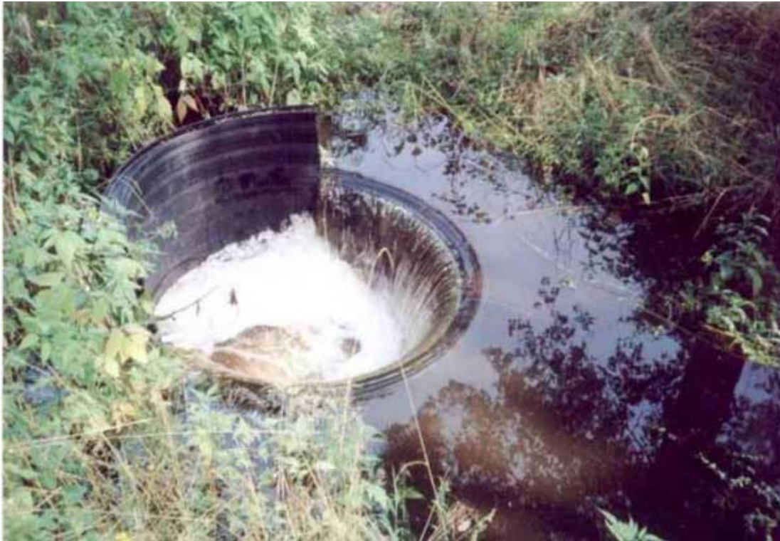
Picture 4. The outflow via the overflow crown of run-off delayer
